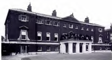
FIGURE 8. Devonshire House. Piccadilly. Demolished. Among aristocratic mansions in London, this townhouse of the dukes of Devonshire was uncommon for being detached instead of terraced. Reproduced by permission of National Monuments Record: RCHME. © Crown Copyright.
